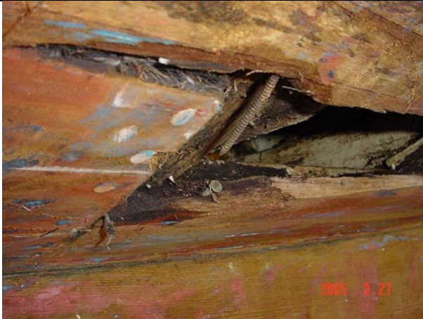
The original hole hacked away with a claw hammer
