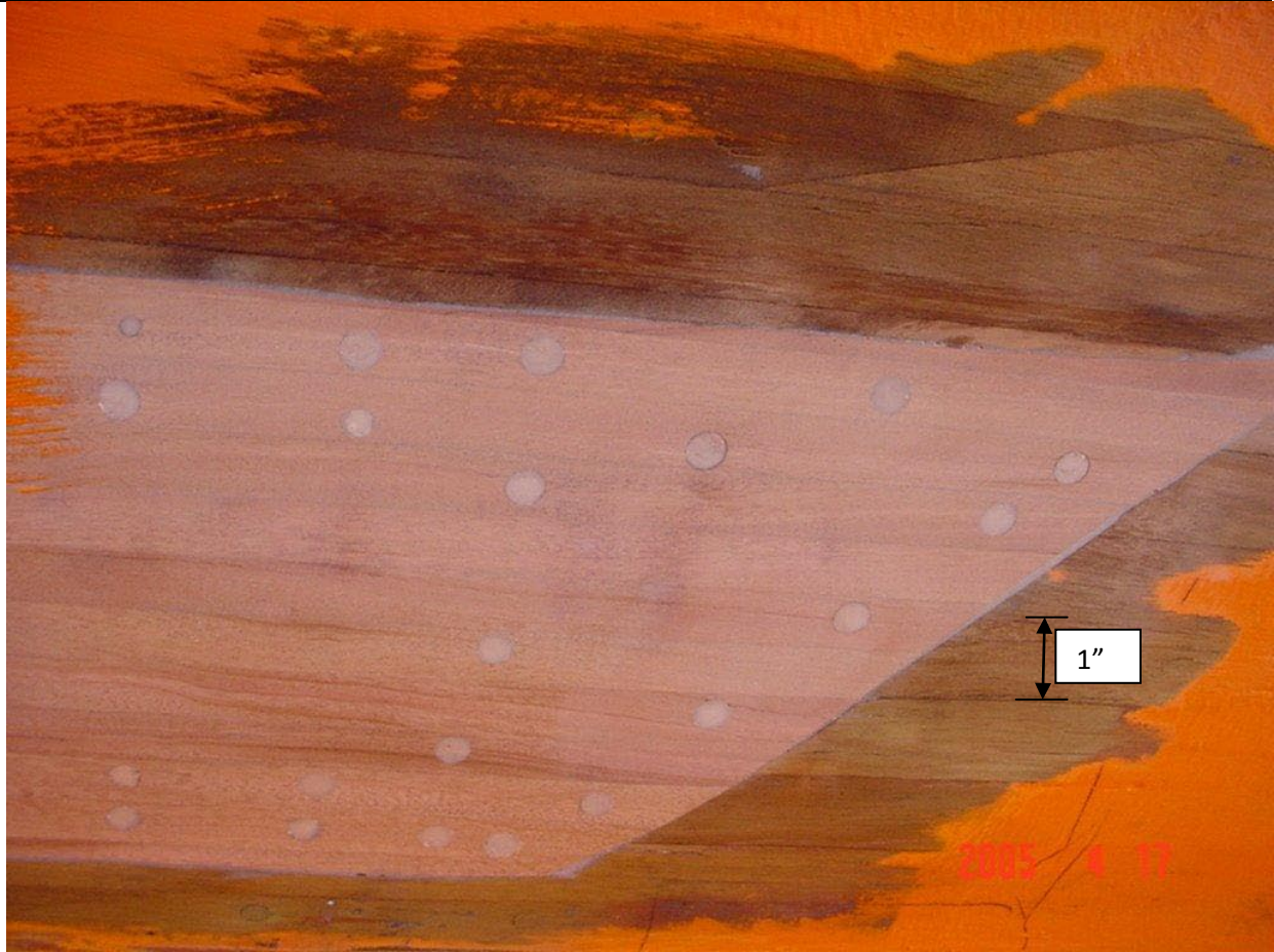
The dutchman after fairing to match surroundings. These joints are nearly imperceptible under the paint. Inspection in 2010 showed no loss of integrity.
